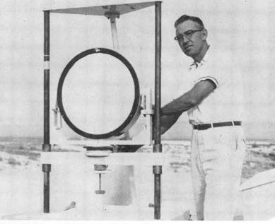
PARABOLIC MIRROR, part of equipment used to collect data on rocket sled tests, is adjusted by Dale Fastle (7244-1). New techniques enable photography showing shock waves and a sharp detailed image of speeding sled on the same piece of film.
